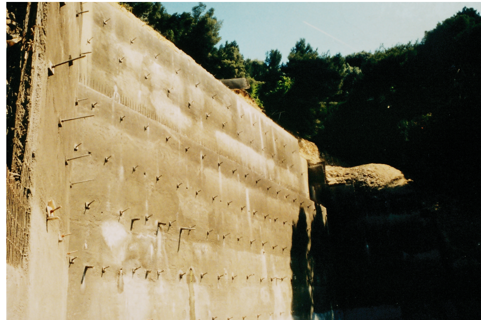
Eugene Corniche Retaining Wall
